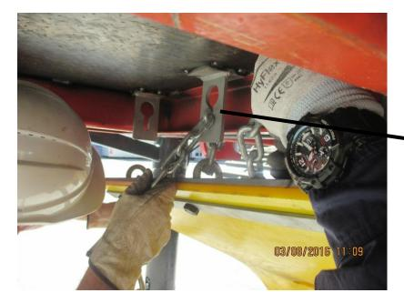
ATTACH 3 CHAINS INTO 3 'T' BRACKETS ADJUSTED TOO HORIZONTAL (SAME NUMBER OF LINKS WILL BE REQUIRED)
